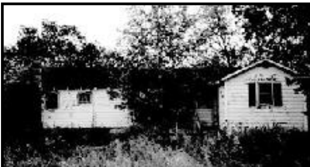
BEFORE: The 236 house before any work had been done (view from N; road is to R of picture)
